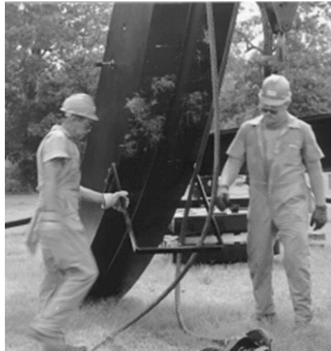
Figure 47: Wireline Bail installation for 120" stroke or greater
