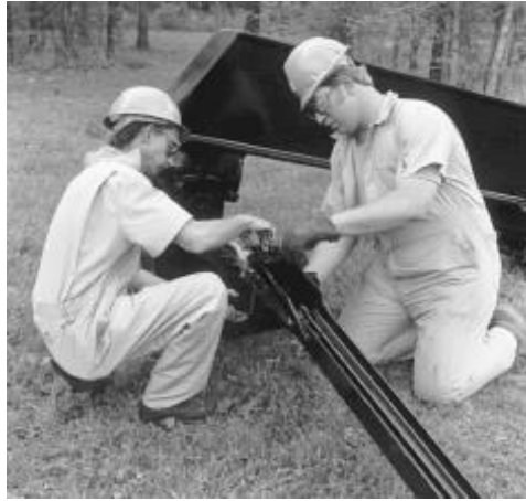
Figure 40: Connection the Pitmans to the Equalizer
