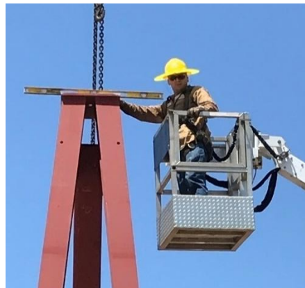
Figure 29: Checking levelness of Samson Post top plate in transverse direction
