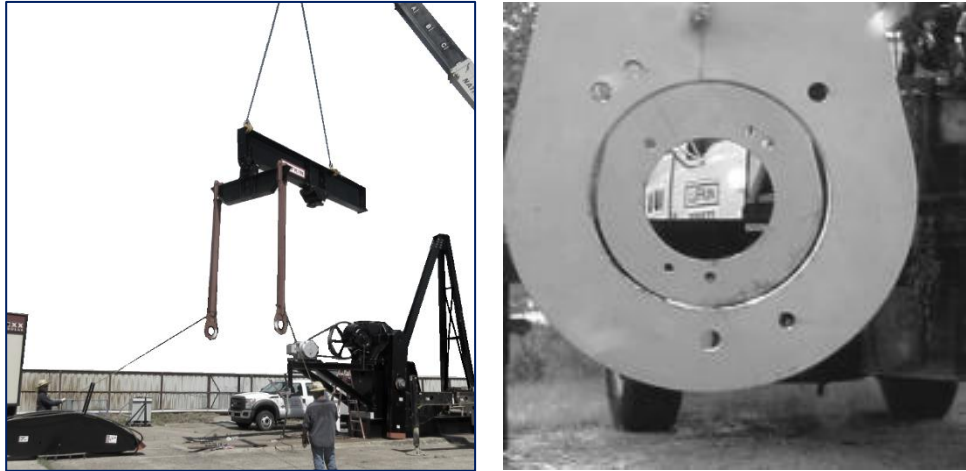
Figure 43: Verifying initial pitman alignment
