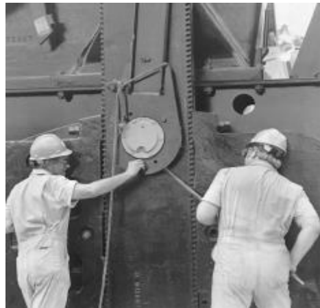
Figure 44: Tightening cap screws joining the Pitman and the Crank Pin Housing
