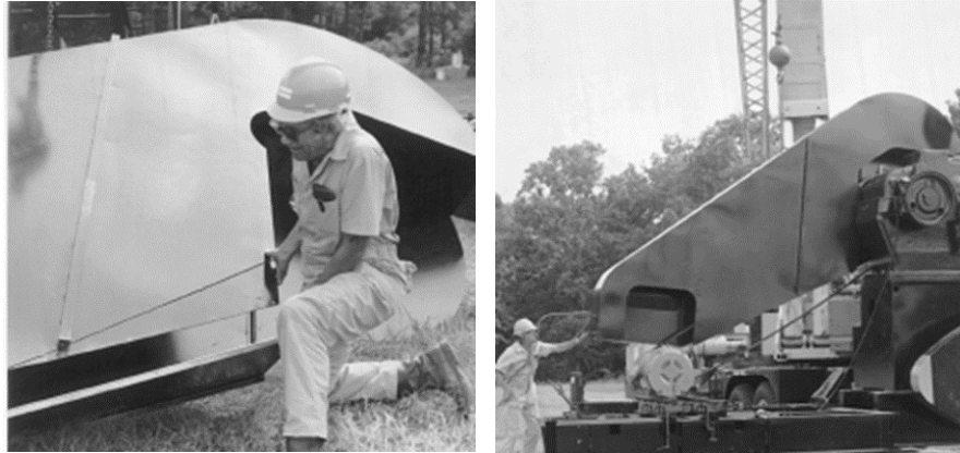
Figure 34: Belt cover installation
