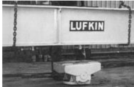
Figure 35: Lifting walking beam for installation to center bearing
