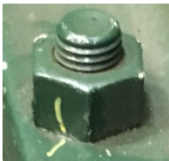
Figure 11: Match mark nut to surface
