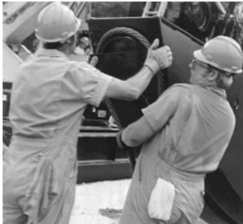
Figure 46: Installing Wireline on Horsehead
