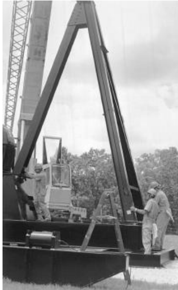
Figure 27: Samson Post assembly during installation
