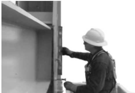
Figure 53: Checking alignment of Horsehead
