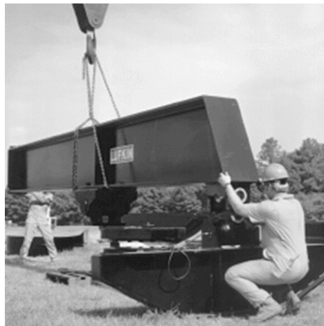
Figure 36: Connecting the Walking Beam to the Equalizer
