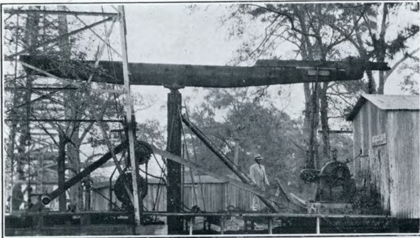
ORIGINAL UNIT FOR HUMBLE CO., GOOSE CREEK, TEXAS —Installed January 1924—still going. Same worm shows little wear, with every evidence of giving service for years to come.
