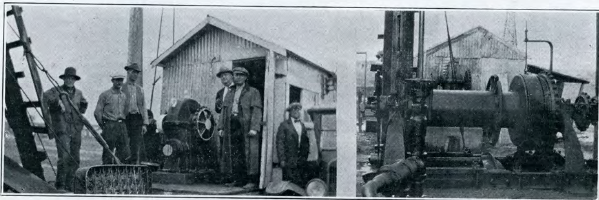
ORIGINAL INSTALLATION, WEWOKA, OKLA.—This Company's General Superintendent, Huey, and Field Superintendent, Gibson, are proud of the results of these units, and of this field, which has not only been a good producer, but is one of the cleanest leases to be found anywhere. Note units painted gray and white.
