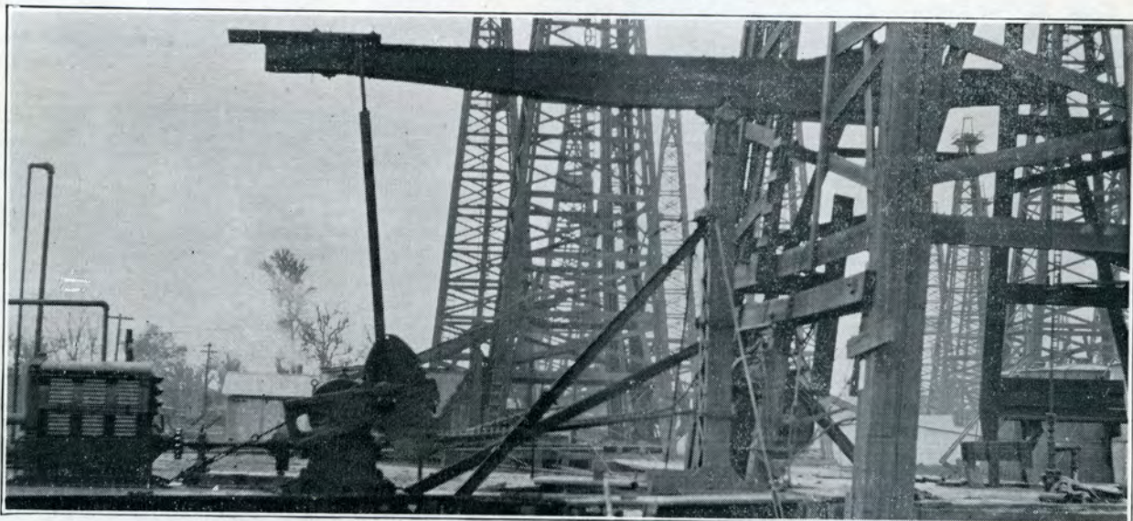
Vacuum Lease, Liberty, 3500'—One of our original units installed with beam balance making 28 strokes, as fast as rig could go, without "whipping" balance weights. Later, rig was equipped with Trout counterbalance, stroke increased to 36 on out hole.
