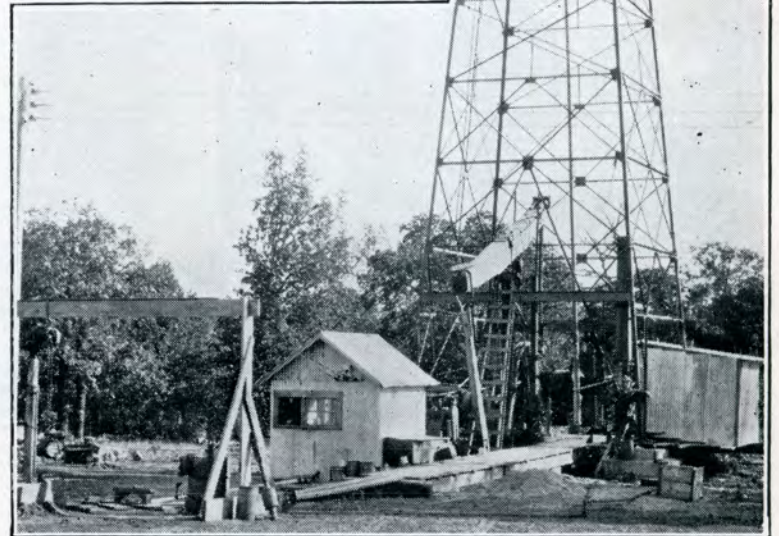
Shaffer O. & R. Co., Davenport, Okla., Drilling in With Electric Motor and Lufkin Units.
