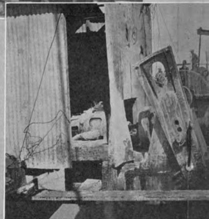
RIO BRAVO WELL #5, SPINDLETOP, THIRTY FEET FROM BURNED WELL. LUFKIN UNIT INTACT. ONLY SALVAGE FROM ENTIRE EQUIPMENT.
