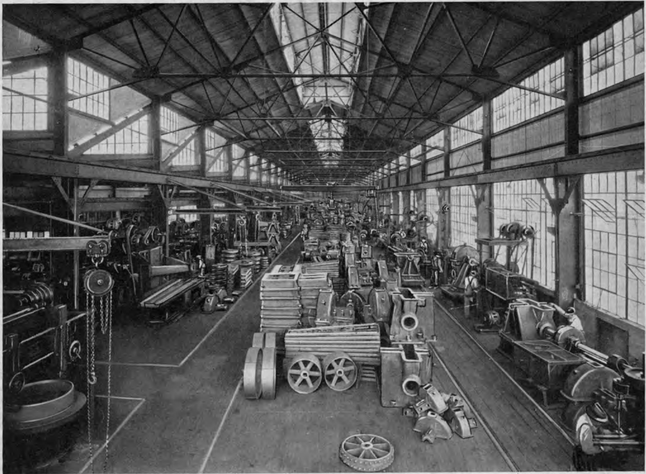
New Machine Shop, 103 feet wide, 386 feet long, where Lufkin Equipment is manufactured by most modern methods. Made strictly to gauges and templates, out of the best materials and with good workmanship.
