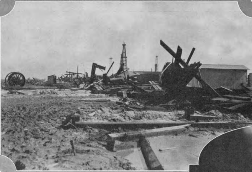
PIERCE JUNCTION WINDSTORM. A ROW OF STANDARD RIGS IN RUINS. NOTE LUFKIN UNITS IN EXTREME END OF PICTURE, UNINJURED.
