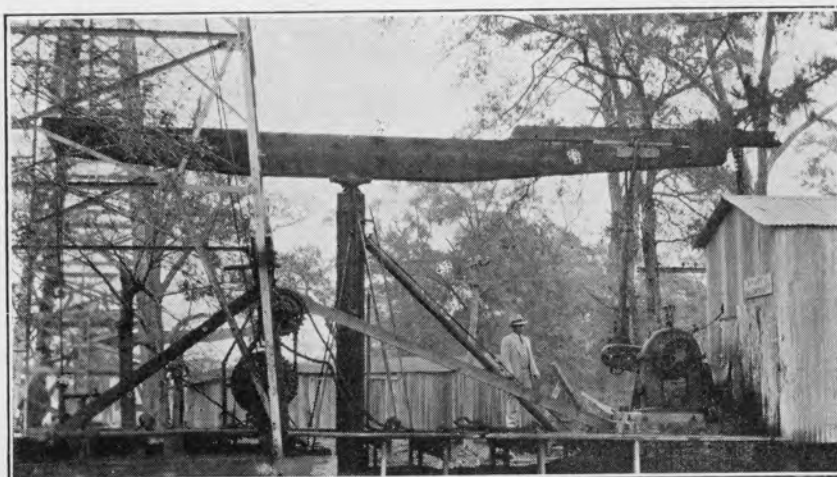
Original installation, Goose Creek, Texas, on Humble Oil & Refining Company's well. Still going with very little signs of wear. This company now has over 100 in use.
