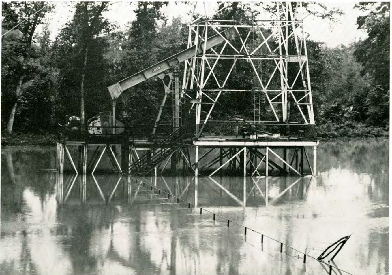
FIGURE 36 Typical installation during high water periods.
