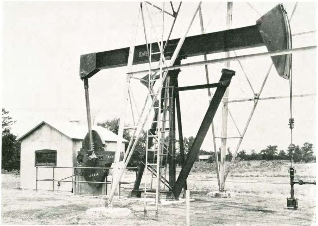
FIGURE 32 Typical Lufkin Single Crank Unit installation.
