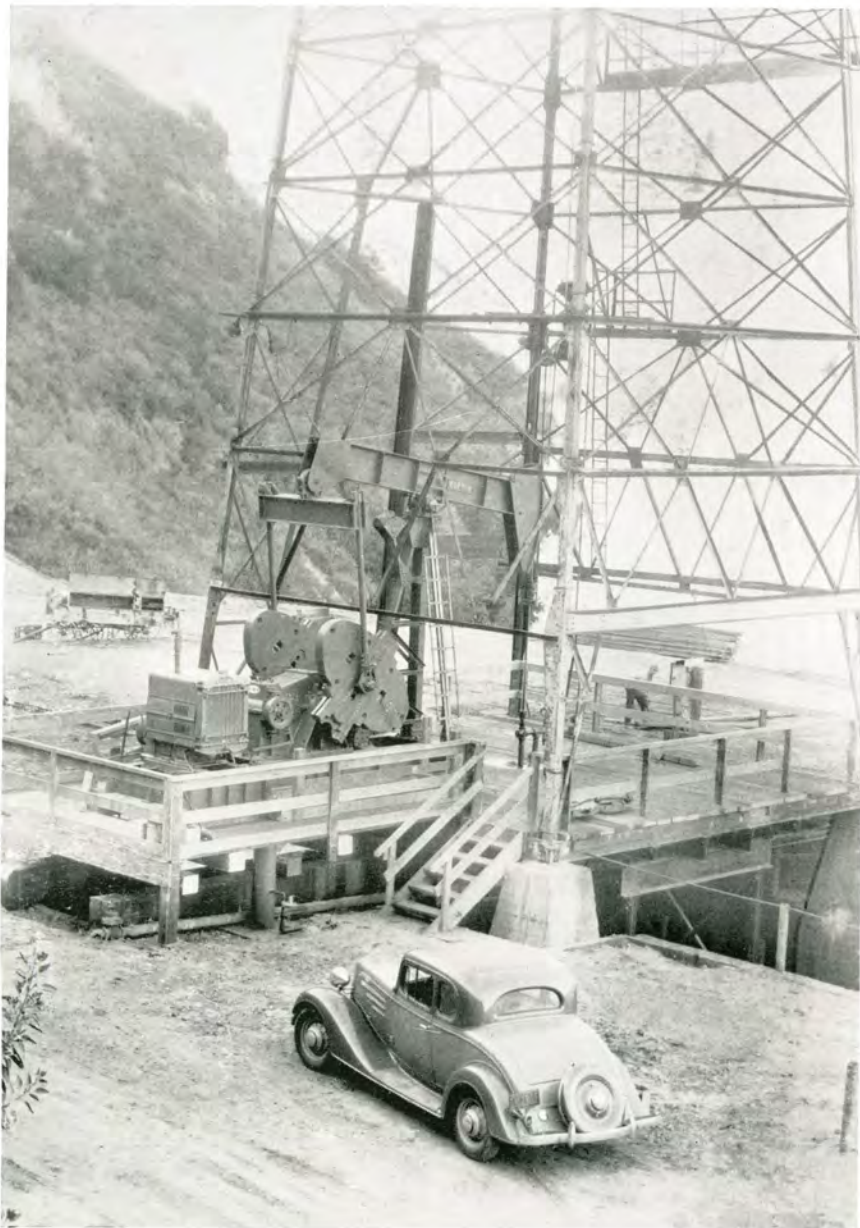
One of many California installations in the heavy deep producing fields where large quantities of fluid are being handled continuously.
