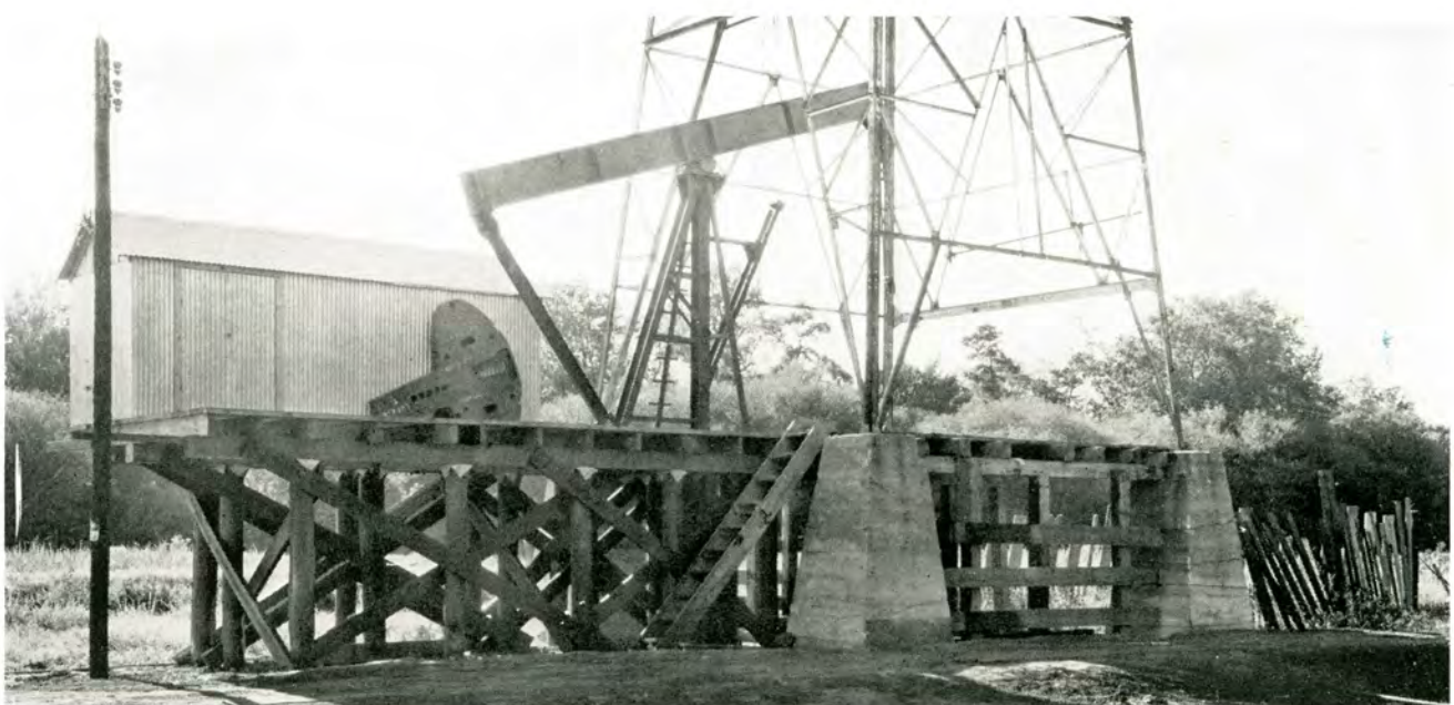
FIGURE 37 Lufkin Single Crank Units and Hoists to individual units are advantageous during either high water or dry summer operations. Portable equipment for pulling is often impracticable for use in connection with this type equipment.
