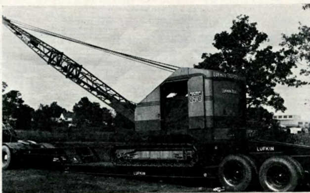
FIGURE 65 Backing trailer to put Goose Neck into rigid position.
