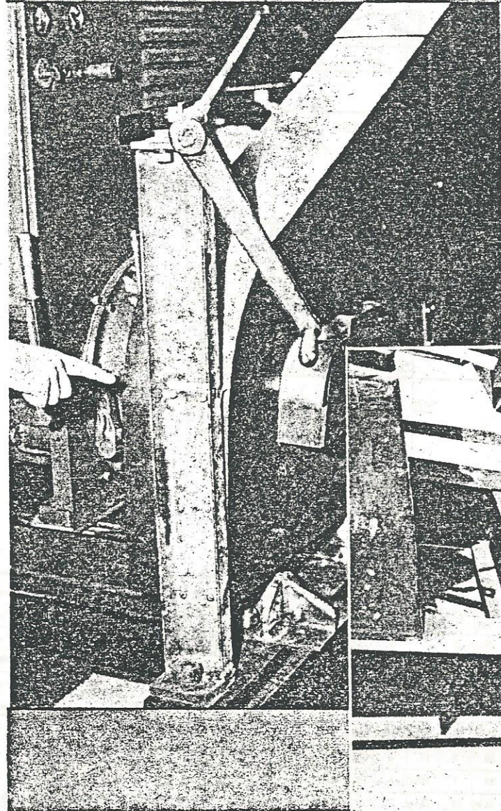
Below: Position of brake lever permits easy accessibility.
